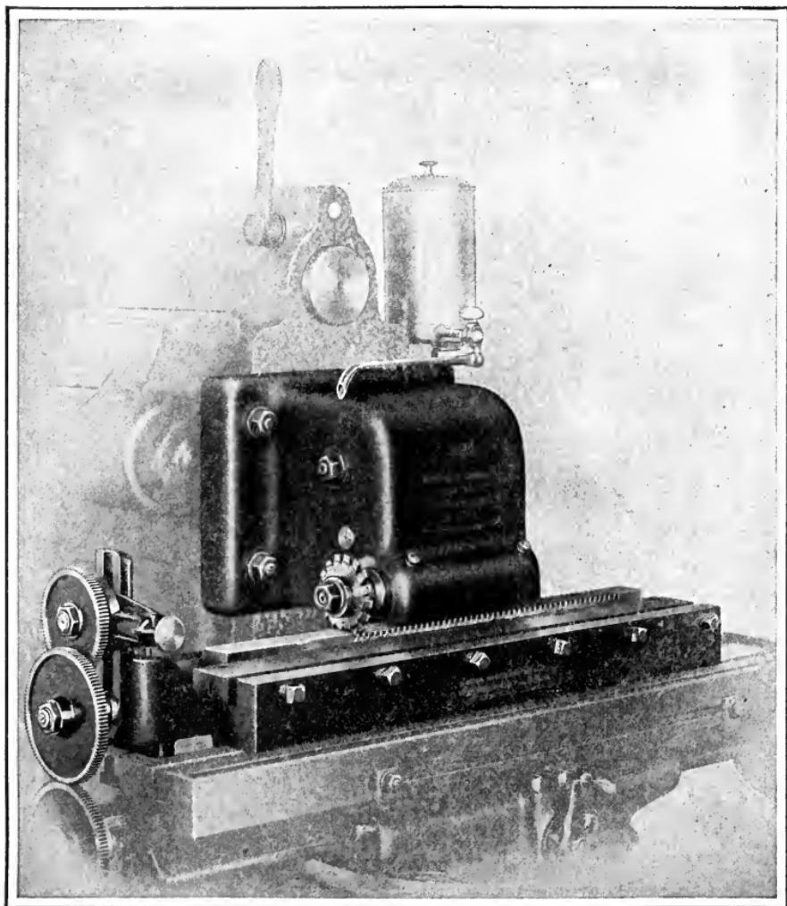
Fig. 246. Rack-Cutting Attachment on Milling Machine
