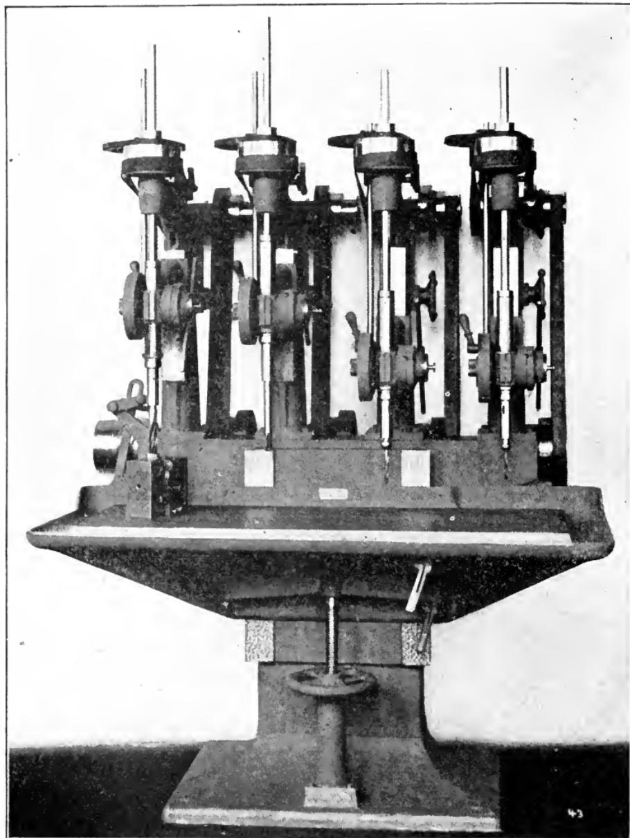
Fig. 349. Four-Spindle High-Speed Ball-Bearing Sensitive Driller
