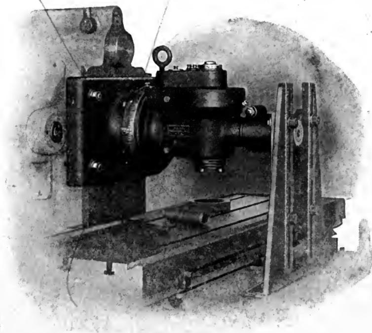
Fig. 229. Vertical Milling Head Attached to Horizontal Milling Machine
