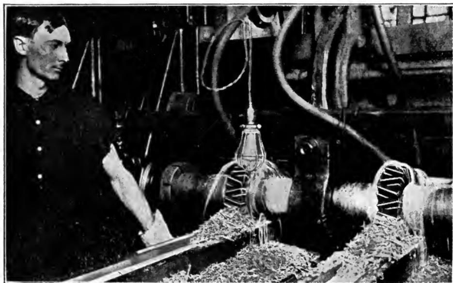
Fig. 347. Ingersoll Horizontal Miller Doing Heavy Milling
