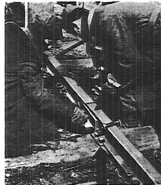
Loosen tie mountings (key, screw, nails) on at least 8 successive ties.
